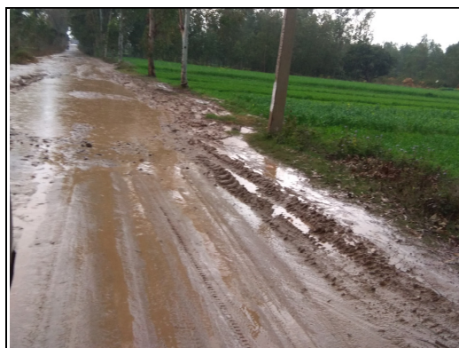
Photograph showing non-existent Sadhaura – Mugalwali road via Rattuwala and Safilpur as on 14 February 2019.
